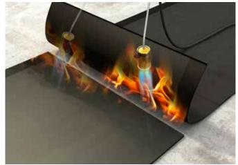
The bonding operations will be facilitated if the sheets are wound around with a rigid plastic tube (HDPE, Ø 12 cm, length 97 cm), which will prevent the ovalisation of the roll during laying, particularly in summer.
