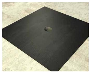
Place the drain and cover with another piece of membrane, half size of the first one. Then proceed with the application of the first layer of the bituminous membrane.
