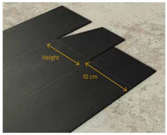
■ Place the membrane on one side of the internal corner.
