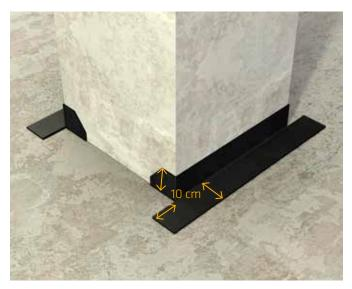
Cut two more pieces of the membrane and place onto the corner.
