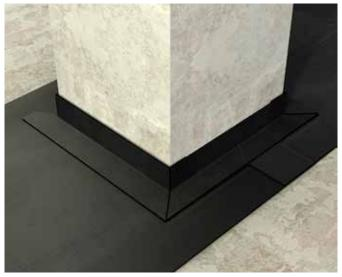
In case of a multilayer system, proceed with the application of the second layer directly onto the first one and finish with the corner details, which must be 5 cm higher than the one below (vertical and horizontal).
