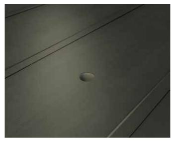
Install the roof vent and bond the base with a piece of the membrane with diameter 10 cm larger.
