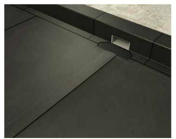
In case of a multilayer system, proceed with the application of the second layer following the same steps of the first layer.
